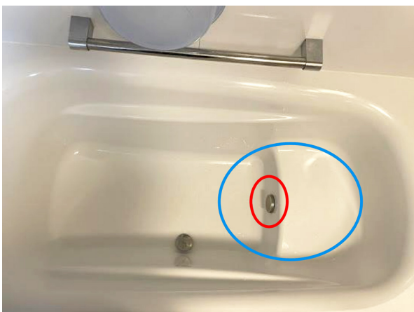
Fig. 3 The bathtub in the patient's house: Cultures of circulation adapter showed the growth of Mycobacterium avium (red circle). The patient was sitting on a bench in the bathtub while the hot water was being poured (blue circle).
